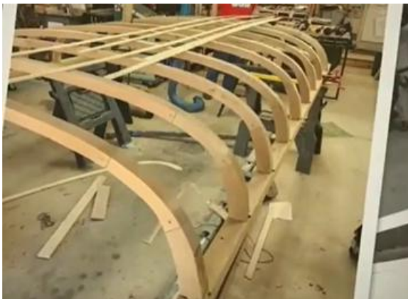
Roof bows installed
