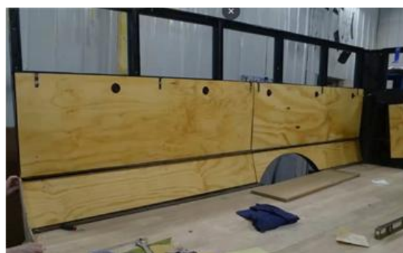
Installation of new interior paneling
