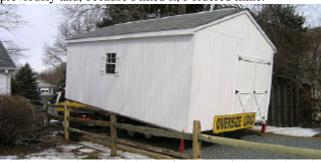
I had prepared a 4 by 4 timber frame one ft. larger than the garage and packed it with ¾in. gravel for drainage. It's quite a sight to see a garage backing up your driveway ready to go. It took only a half hour to position the garage, and load the advance vehicle with the warning sign onto the trailer for the return trip. Hank Dubois assisted in aligning the garage. Eric, Eli and Nate Sumner missed the delivery but arrived in time to give the garage a final inspection.
