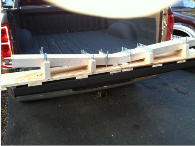
Front header pieces ready to have finger joints cut.
