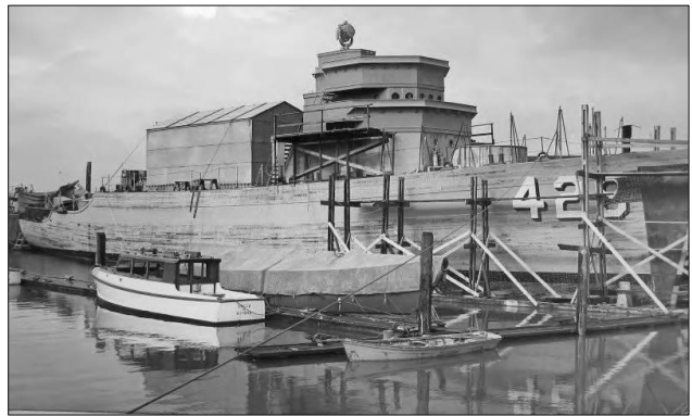
This picture of the USS Dash under construction clearly shows the ship's wooden hull.
