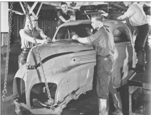
Workers wet block sand the body on this '38 Lincoln Zephyr body that appears to be a 3 Window Coupe. See Coupe image on page 2.
