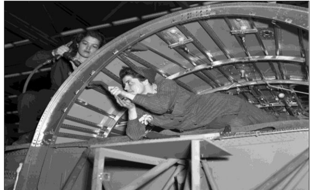
This picture, taken at Willow Run, clearly shows both the riveter outside the B-24 fuselage and the woman inside holding the bucking bar. The rivet was obviously inserted from inside the fuselage and then peened from the outside.
