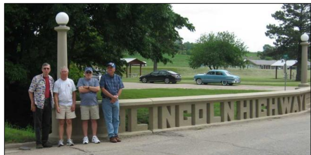
This is a cool original bridge built in 1915 in Tama, Iowa. – Bill Simons
