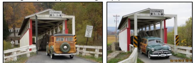
Woodies and the wooden bridge.
