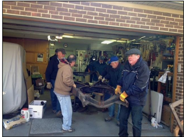
Moving the frame outside for repair work before sending it out for blasting and paint also freed up room for Dave to work on the running gear and other parts. You never can have TOO MUCH garage space!
