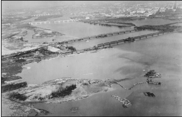
Dredging at Gravelly Point began in 1938. The half completed Memorial Bridge can be seen crossing the Potomac in the upper part of the image.
