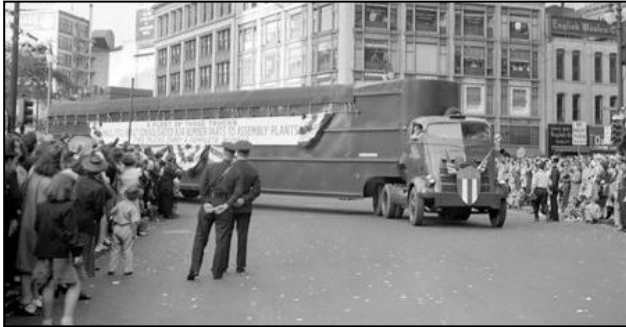
This pictured shows the dual-engined rig negotiating a corner hauling one of the specially built 60 foot trailers.
