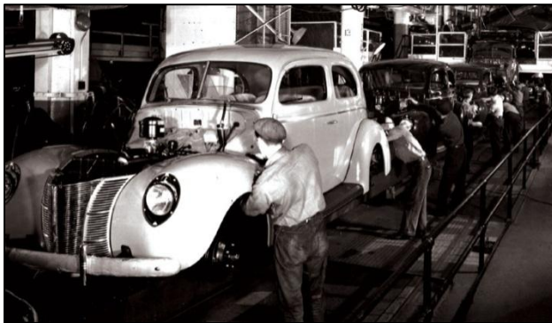
Front fenders are bolt up to this 1940 Deluxe Tudor right after the body drop.
