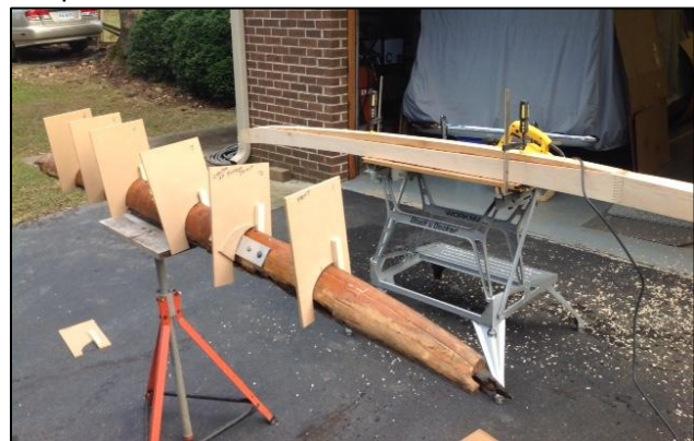
New top side beam takes shape in the background.
