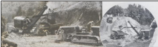
Ford COE dump trucks were used by Pennsylvania Turnpike contractor Nello L. Teer. Ford News , October 1940 image.
