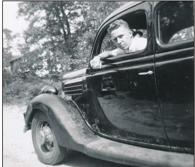
Before the checkerboard hood louvers.
