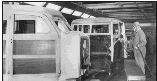
The sheet metal was masked off before the varnish was sprayed.
