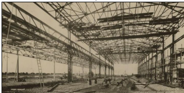
The Geelong assembly plant under construction in 1925.
