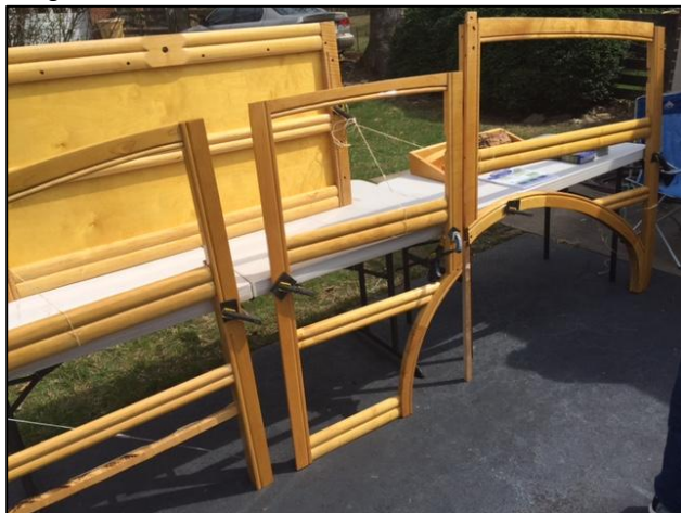
All the wood is varnished and ready to be re-installed after the paint work is completed.
