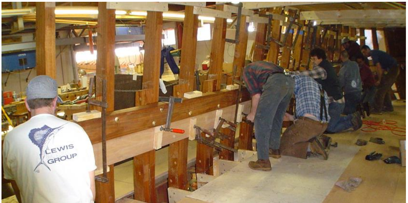
Workers clamping steamed wood into place.
