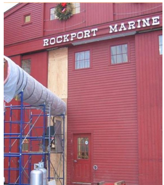
Steaming took place in a specially constructed "oven."
