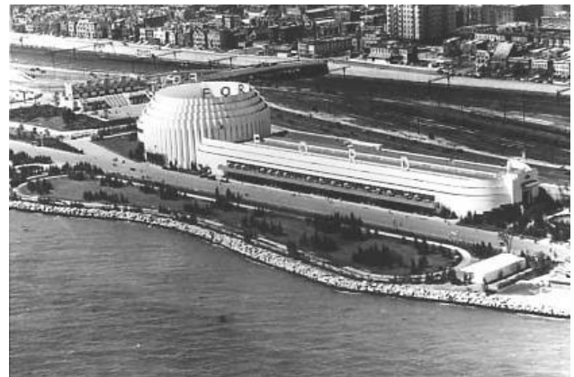
The Ford Building and Rotunda with Roads of the World in the foreground.
