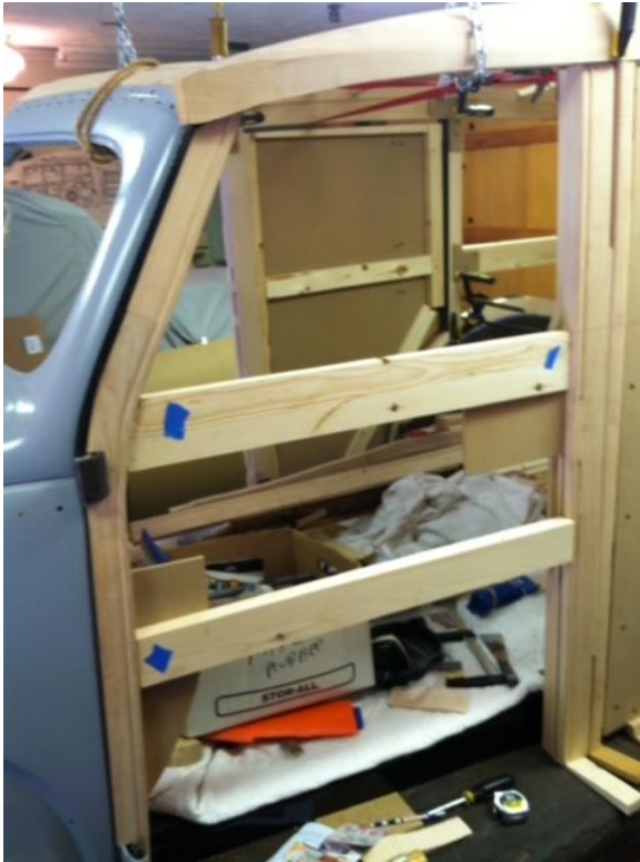
The front and rear door posts are in place. You can see the slot in the rear post for the panel insert.
