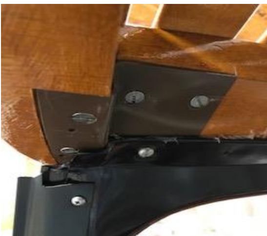
The bracket successfully installed.
