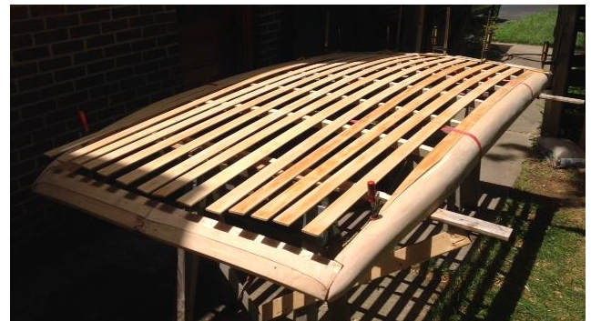
The basswood slats being fitted to the roof assembly.
