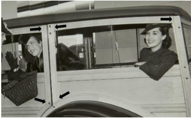
Just a few of the lap joints on a '39 Ford Woodie.
