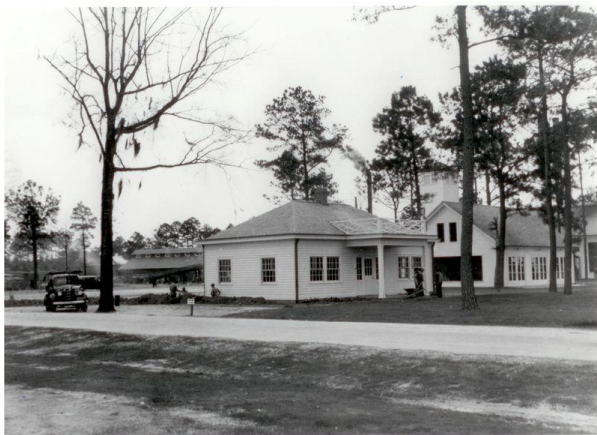
The Plantation Office housed offices for the supervisor, payroll clerk, and accountant
