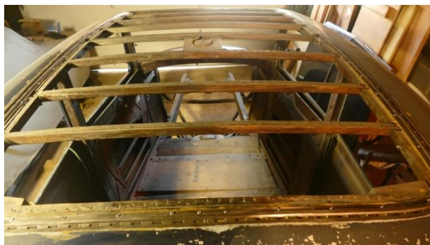
Top Wood Installed
