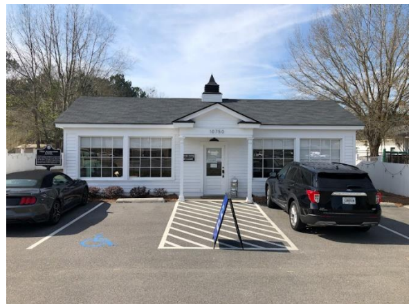
Ford Bakery Building and Richmond Hill Visitors Center
