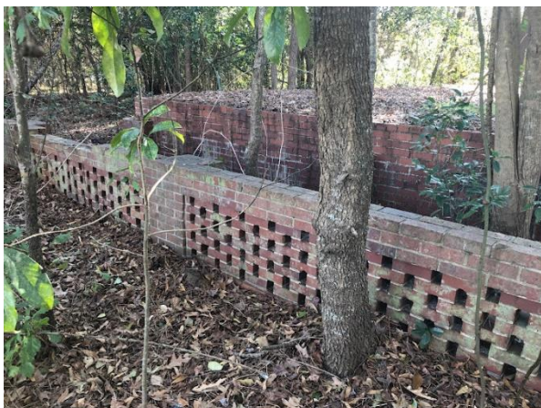
All that remains of the Ice Plant is the foundation
