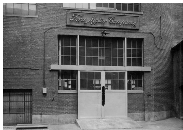
Rear Vehicle Service Entrance
