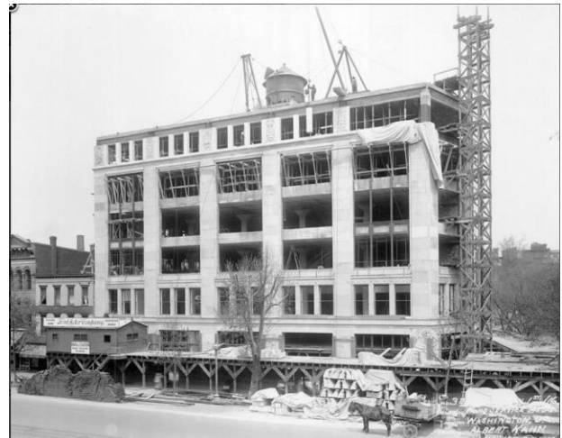
The Pennsylvania Avenue façade – 1 March 1916
