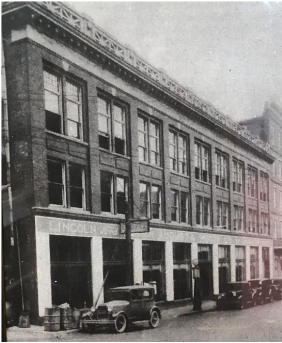
The same building in the 1920s.
